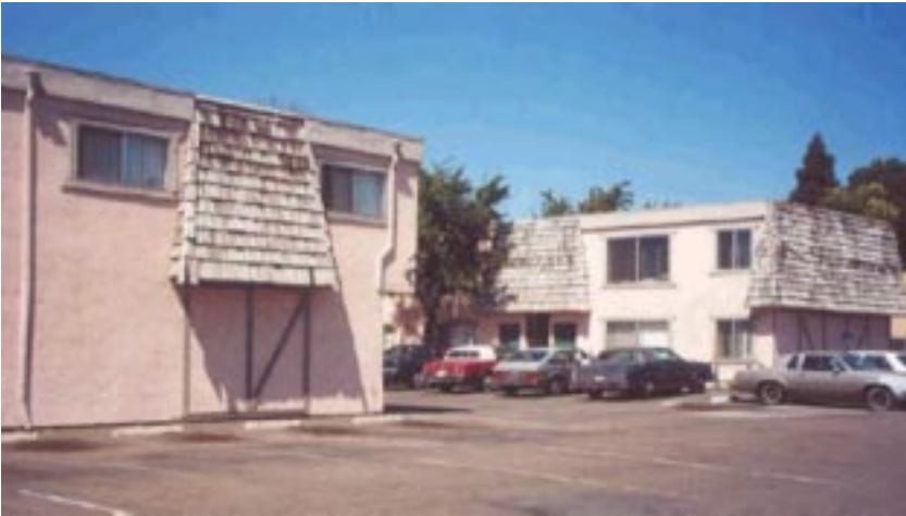
The site of St. Regis Park before its rehabilitation.
